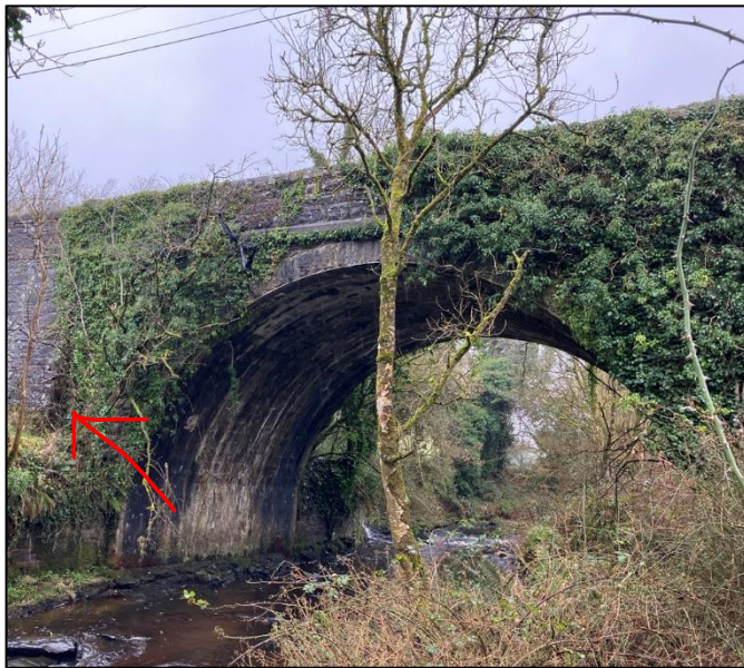
Plate 4-8. Single-arch stone bridge. The arrow indicates the vertical crevice.
